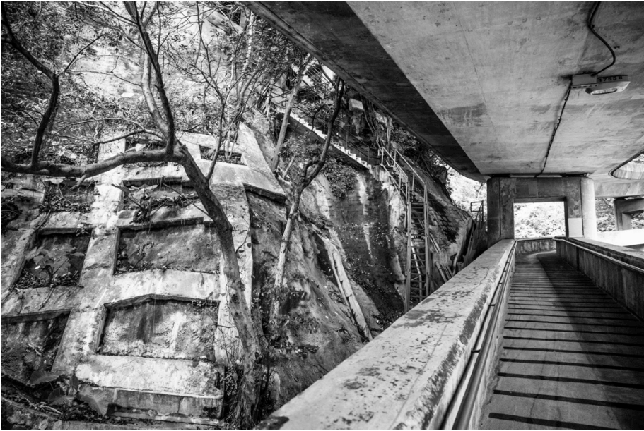
Figure 2. Example of a Hong Kong “registered slope” stabilization technique
